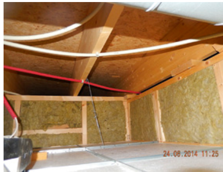
Hulrom over himling uten sprinkler
