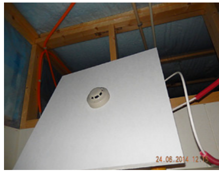
Detektor i himling funnet over himling.
